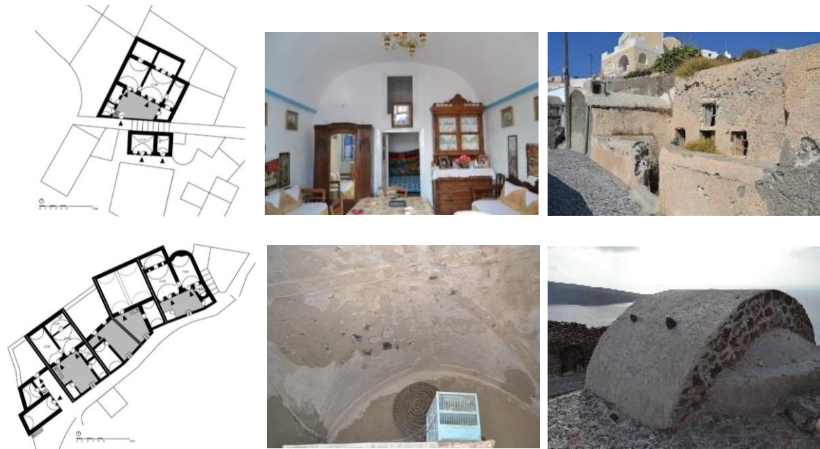
Figure 2: The spiti vaulted house of Thirasia island (Santorini, Greece). Plan of the houses in Potamos (top left) and Manolas (bottom left) and respective exterior and interior with barrel and groin vaults (right). (Author's drawing and photos)
